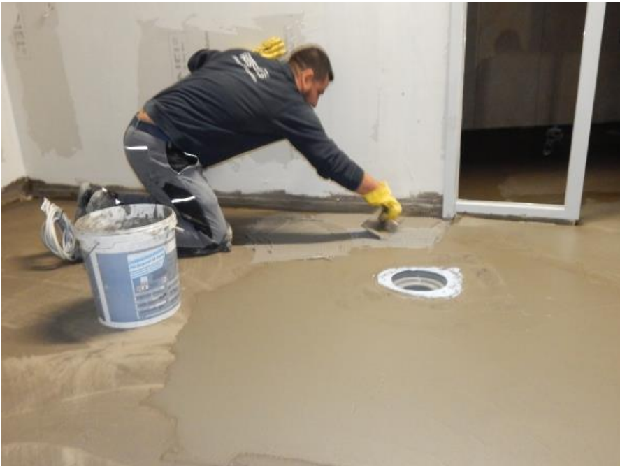
The tile layers used PCI Seccoral 2K Rapid for the central relaxation pool in the Oriental Bath. ( Link to high-resolution photo, ©PCI Augsburg GmbH)
