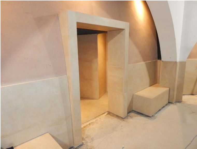
Each of the benches on all sides of the pool surround appears to be made from a single thick slab of natural stone. ( Link to high-resolution photo, ©PCI Augsburg GmbH)
